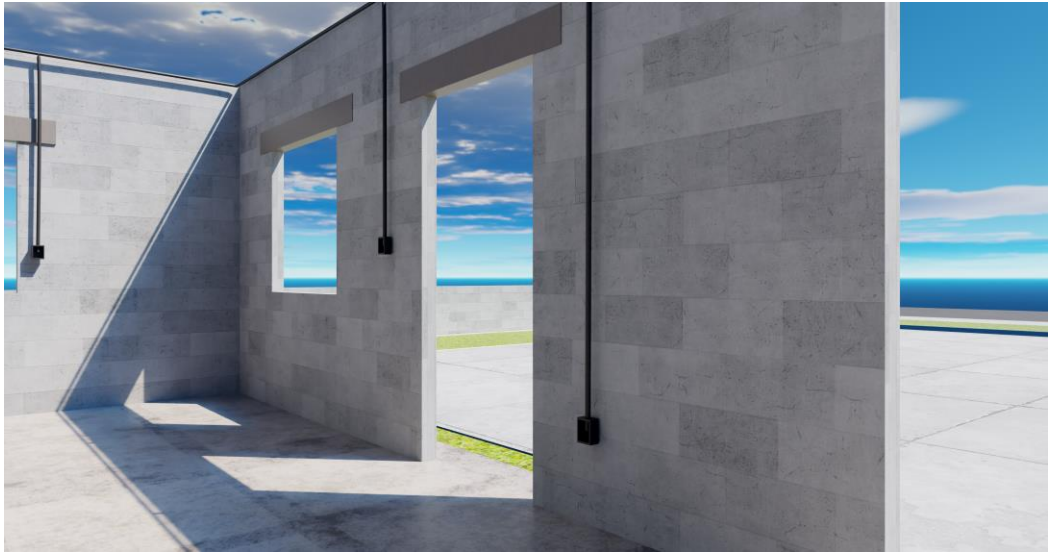
Figure 11 - Electrical conduit being placed
