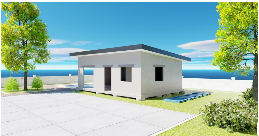
Figure 9 - Weathertight building. Roof, windows, doors, and building wrap all installed
