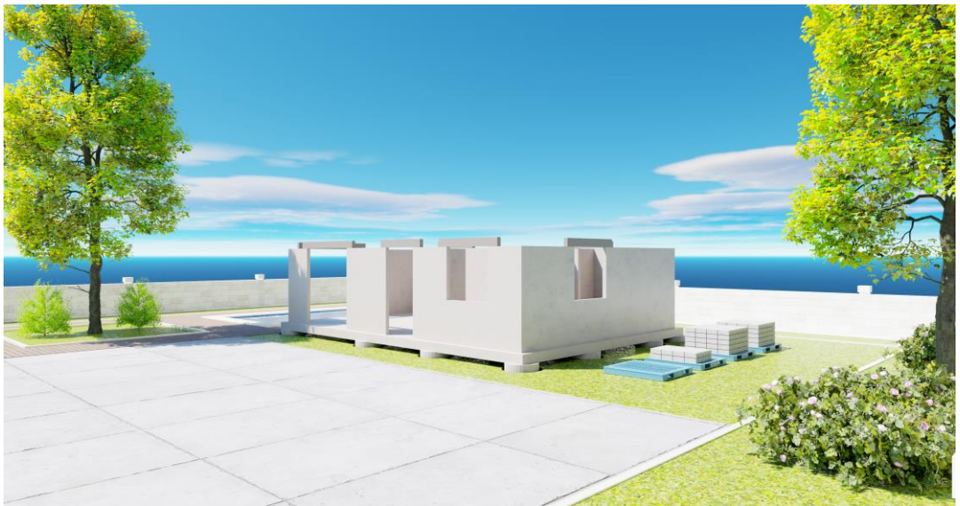
Figure 8 - Window and door headers are placed
